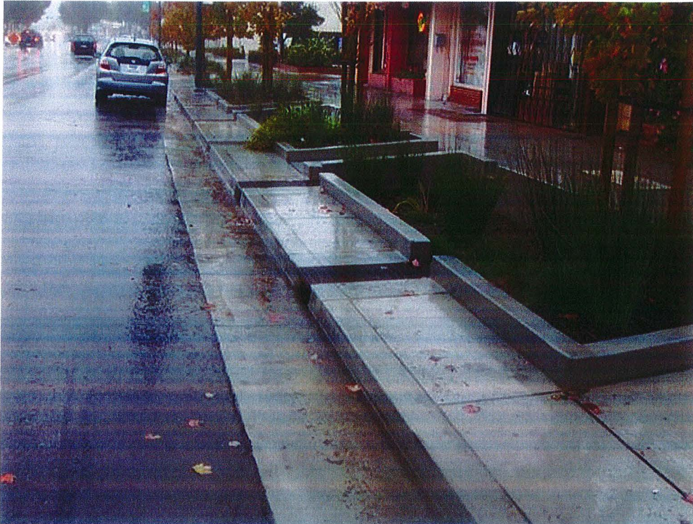
Figure 1: Off-line system in El Cerrito where low flow is diverted to the sidewalk planter and high flows continue down the gutter.
