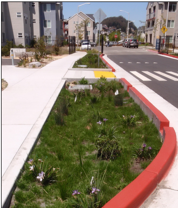
Figure B-10. Curb Extension. In addition to reducing the street width and shortening the length of street crossings for pedestrians, curb extensions, or “bulbouts,” such as this example in Albany, also provide space for GI facilities.
