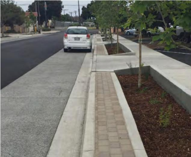
*Porous Concrete Parking Lane, City of Ventura CA (<https://nacto.org/publication/urban-street-stormwater-guide/stormwater-elements/green-stormwater-elements/permeable-pavement/>)*
