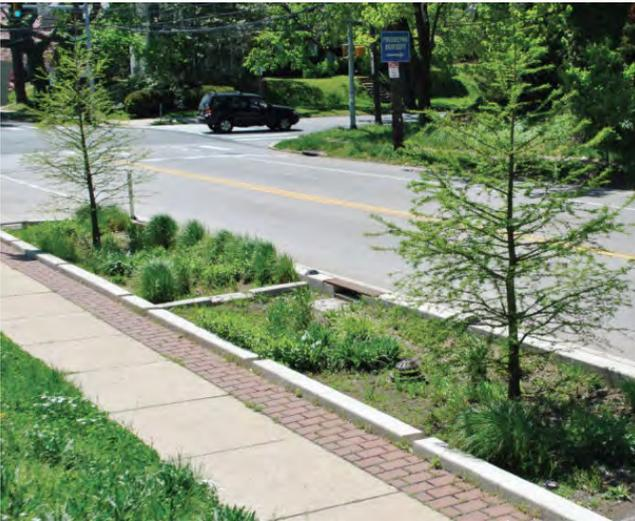
*Bioretention bulbout in Philadelphia, PA (<https://nacto.org/publication/urban-street-stormwater-guide/stormwater-elements/green-infrastructure-configurations/stormwater-curb-extension/>)*
