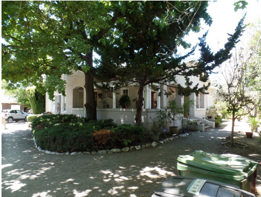
Figure 4. Gravel driveway leading to garage at left and walkway leading to entrance at the primary east facade at right (Garavaglia Architecture, Inc.)
