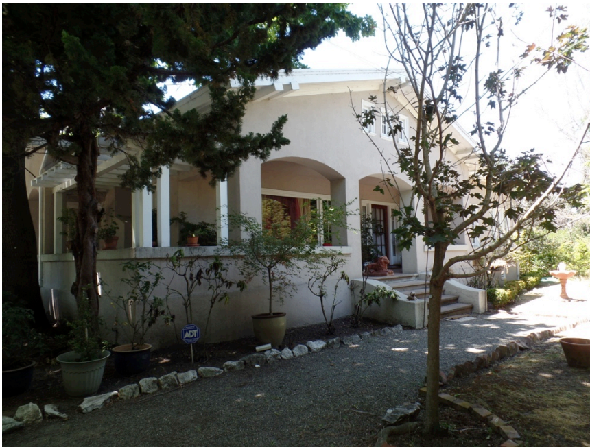
Figure 7. Covered front porch at east facade, looking northwest (Garavaglia Architecture, Inc.)
