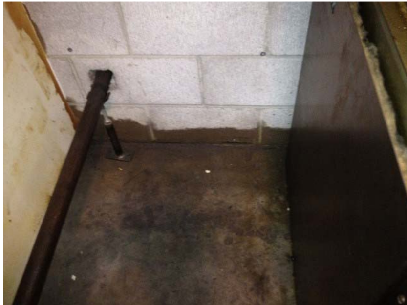
Photo 2. View of concrete floor with apparent staining inside basement-level elevator machine room. Photograph taken on October 21, 2014.
