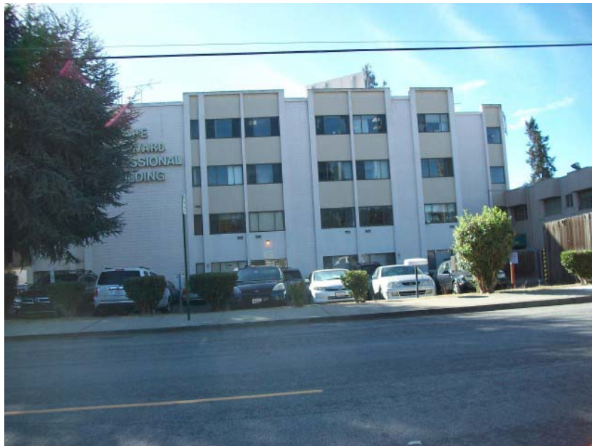
Photo 2. View from McKeever Avenue, looking south, of subject property four-story building. Photograph taken on October 21, 2014.
