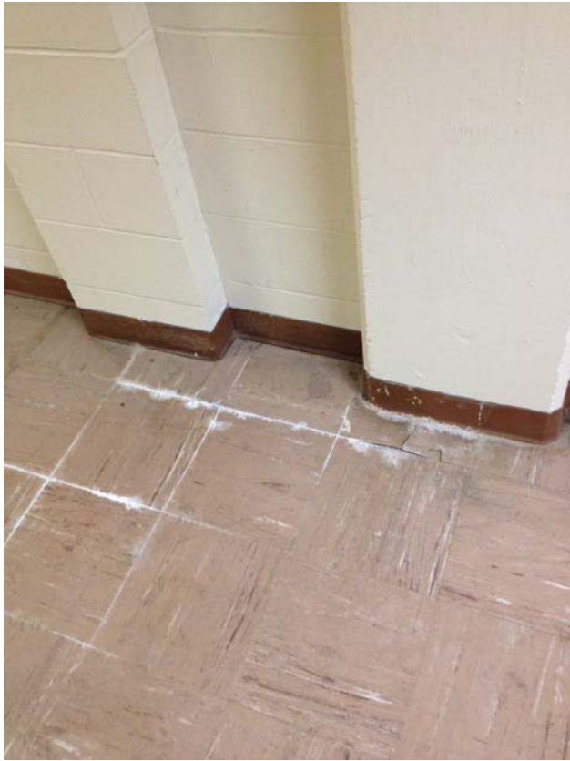
Photo 1. View of possible water intrusion area in basement floor. Photograph taken on October 21, 2014.
