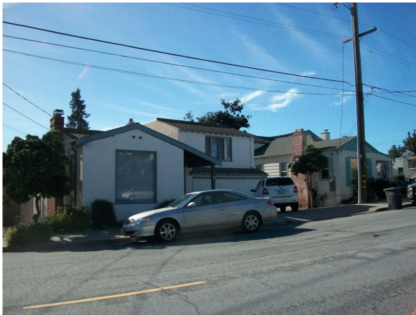
Photo 1. View looking south of 1013 McKeever Avenue. Photograph taken on October 21, 2014.
