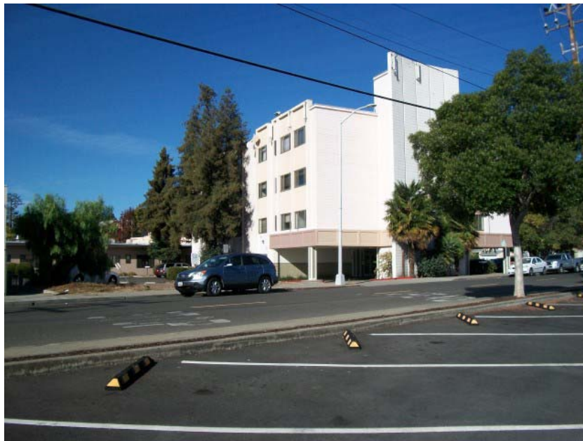
Photo 1. View from Maple Court, looking northwest, of subject property four-story building. Photograph taken on October 21, 2014.
