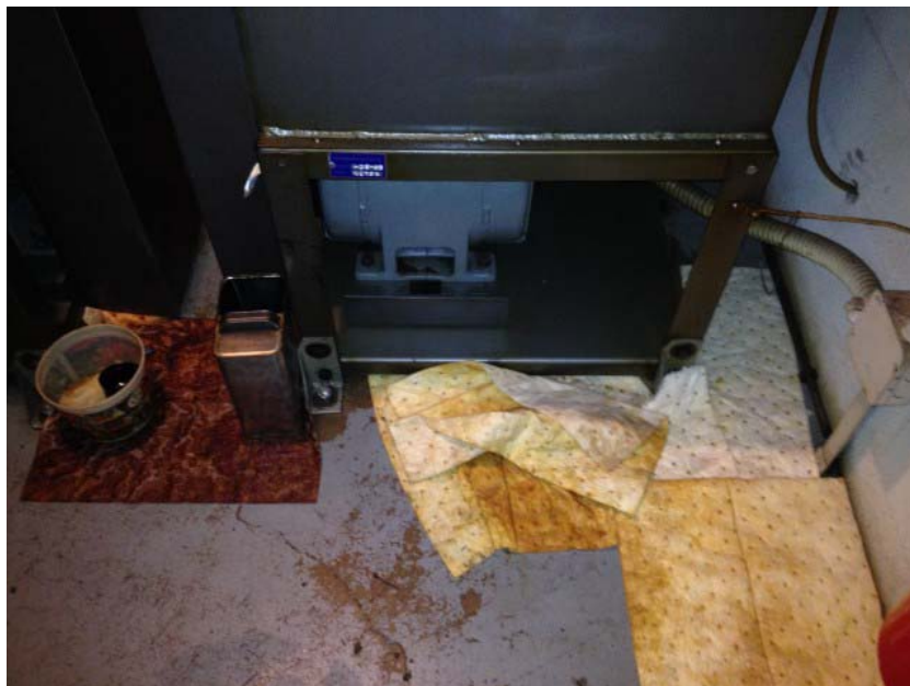
Photo 1. View inside basement-level elevator machine room; absorbant pads, staining and leakage of hydraulic fluid apparent on concrete floor. Photograph taken on October 21, 2014.
