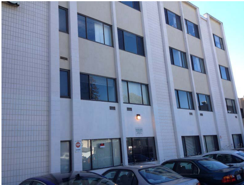
Photo 2. View of northern side of subject property four-story building. Photograph taken on October 21, 2014.
