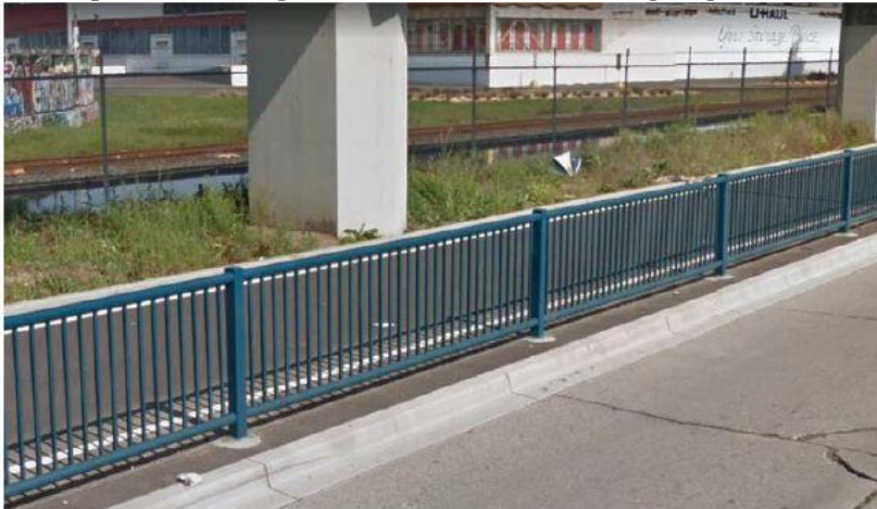
Example of existing rail fence character along Segment 7A of the Greenway project
