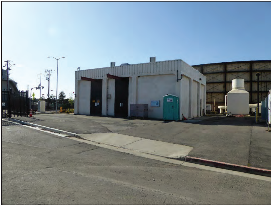
Photograph 38. Building 34 (Headworks) with Structure 1 (West Trickling Filter, background right); camera facing southeast, April 21, 2017.
