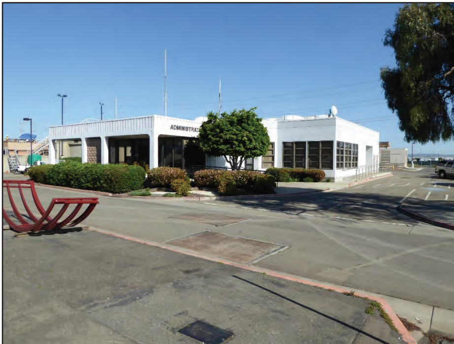
Photograph 19. South and west sides of Building 17 (Operations Building); camera facing northwest, April 21, 2017.
