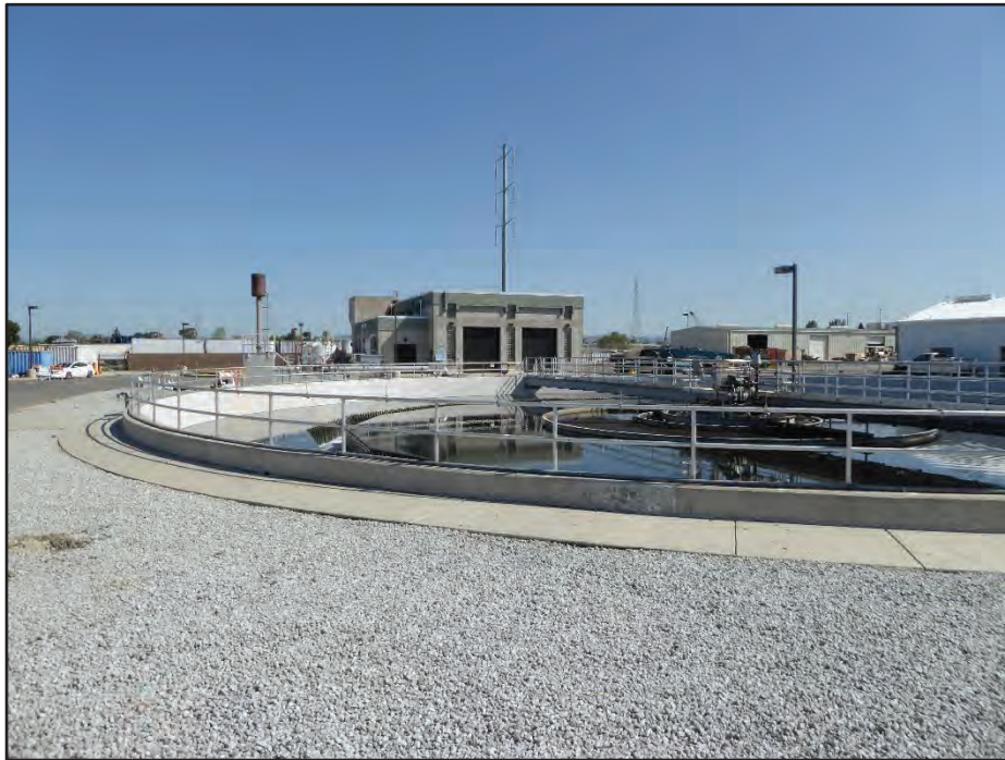
Photograph 50. Structure 47 (Final Clarifier 1, foreground) with Building 44 (Solids Thickening Building, background center), Building 37 (Warehouse, background center right), and Building 27 (Maintenance and Electrical Shop, background far right); camera facing northeast, April 21, 2017.
