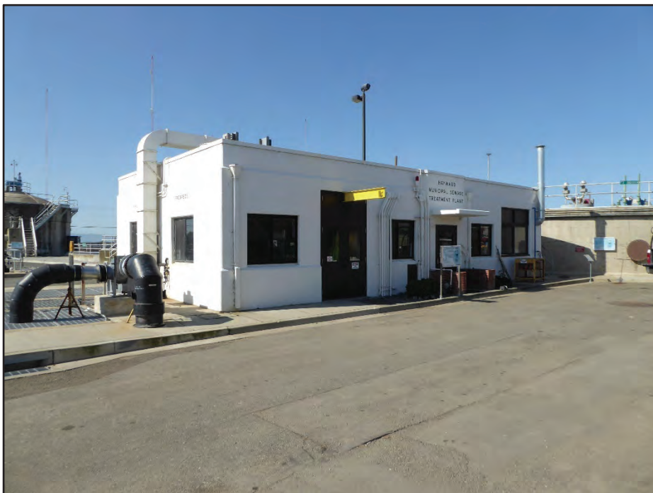
Photograph 9. North and east sides of Building 8; camera facing southwest, April 21, 2017.
