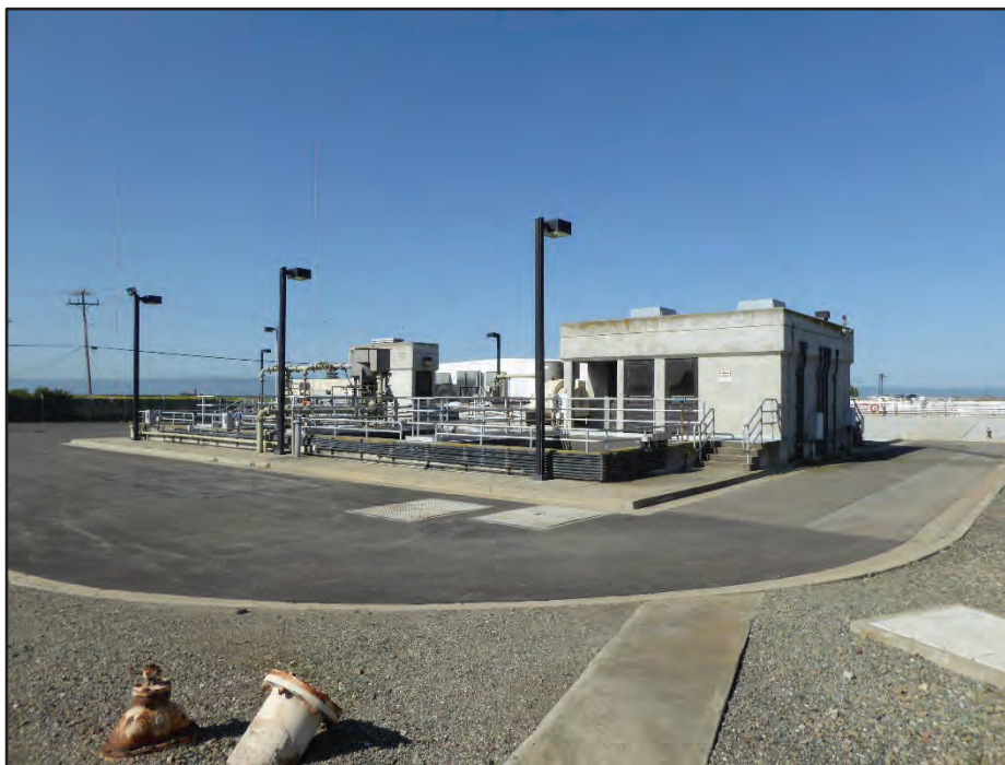
Photograph 32. Structure 29 (Fluid Bed Reactor); camera facing southwest, April 21, 2017.
