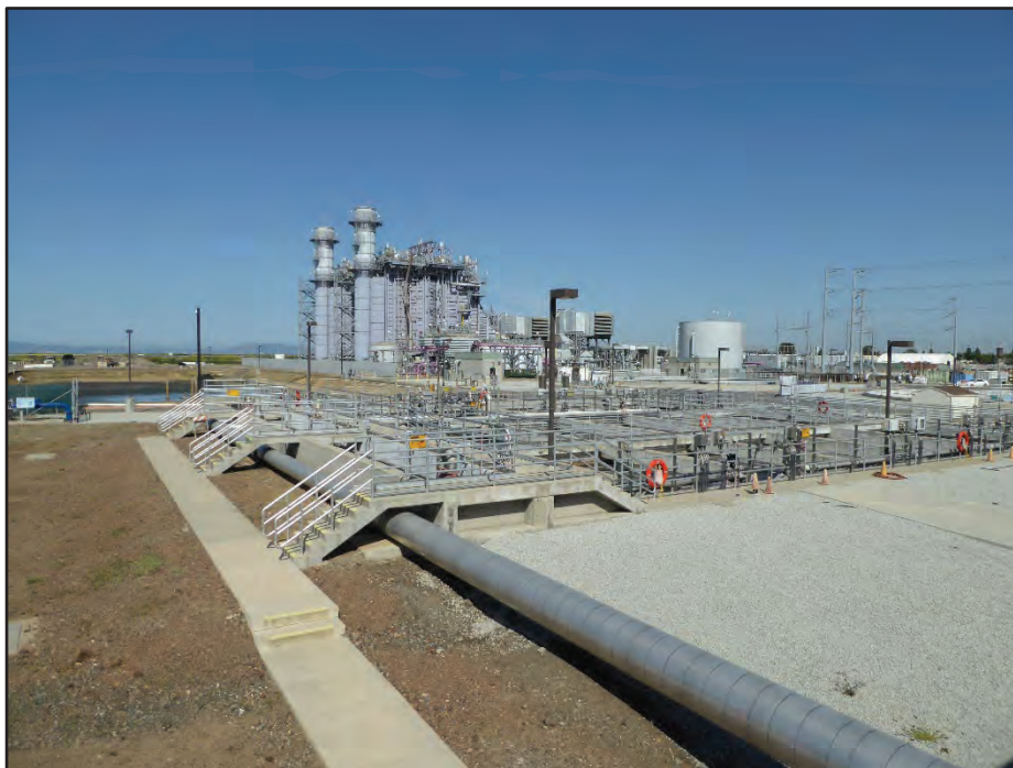
Photograph 35. Structure 32 (Solids Contact Basins) with the Calpine Energy facility in the background; camera facing northwest, April 21, 2017.
