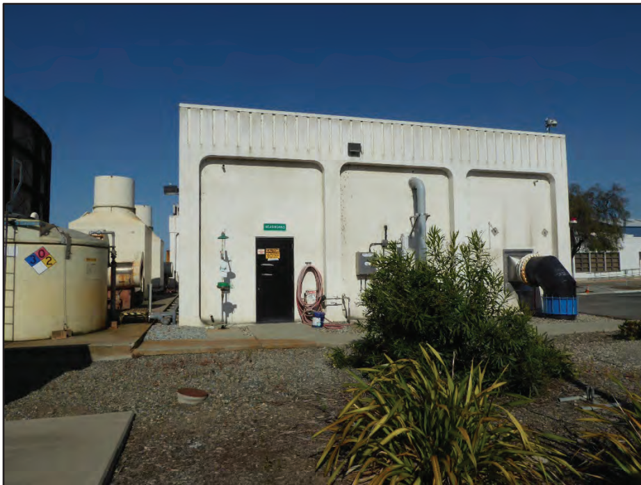
Photograph 39. East side of Building 34; camera facing west, April 21, 2017.
