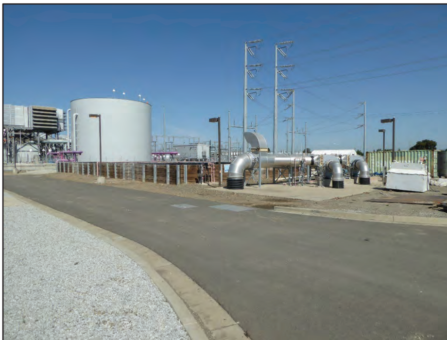
Photograph 48. Structure 45 (West Bio Filter); camera facing northwest, April 21, 2017.
