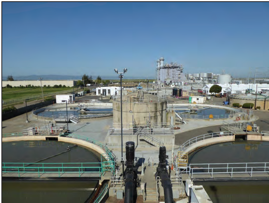
Photograph 5. Structure 2 (North Primary Clarifier, bottom right), Structure 3 (South Primary Clarifier, bottom left), Structure 4 (Northwest Primary Clarifier, center right), Structure 5 (Southwest Primary Clarifier, center left), Structure 6 (South Vacuator, center). The Calpine Energy facility is in the distance, camera facing west, April 21, 2017.
