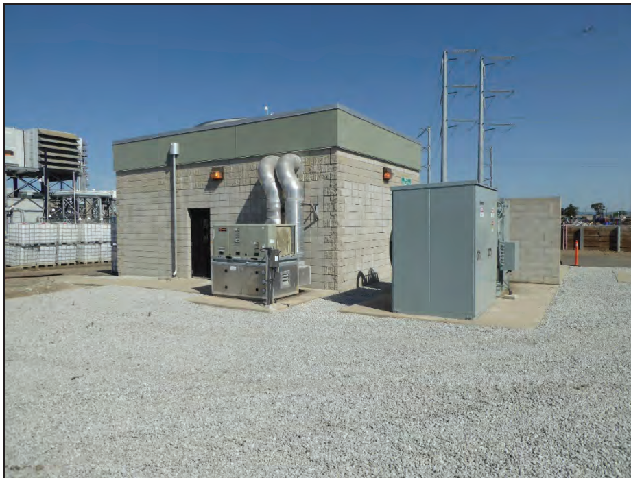
Photograph 49. Building 46 (West Substation); camera facing northwest, April 21, 2017.
