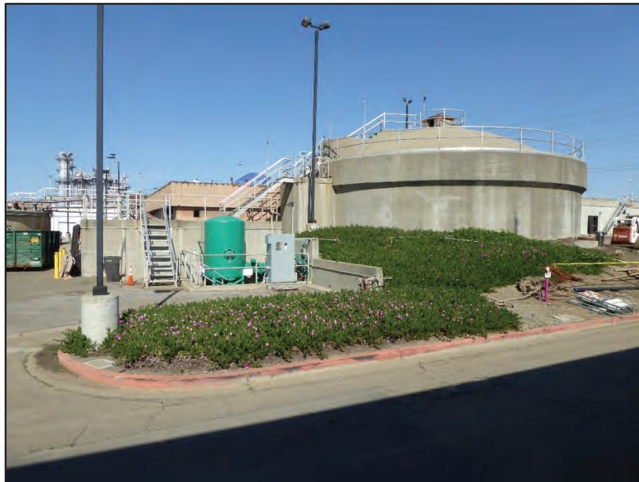
Photograph 15. Structure 13 (North Vacuator); camera facing northwest, April 21, 2017.
