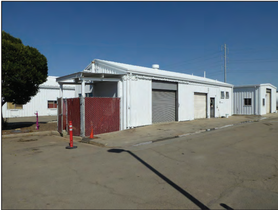
Photograph 18. South and east sides of Building 16, with Structure 21 (Gasoline Pump, south side of Building 16); camera facing northwest, April 21, 2017.
