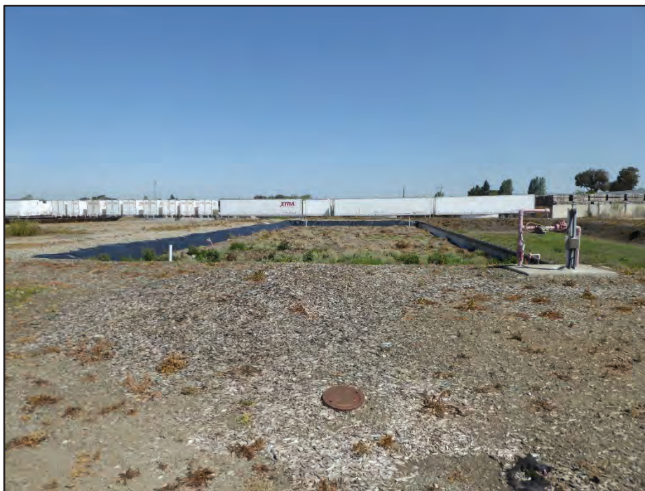
Photograph 46. Structure 43 (East Biofilter); camera facing north; April 21, 2017.
