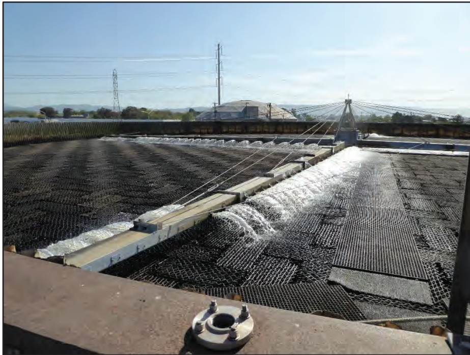
Photograph 4. Detail view of Structure 1 roof / trickling equipment; camera facing northeast, April 21, 2017.
