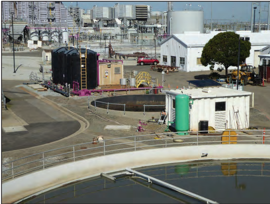
Photograph 16. Structure 14 (Sludge Conditioning Tank, center), with Structure 15 (Water Reclamation Station, center background), Building 20 (Air Compressor Building, center right), Structure 4 (Northwest Primary Clarifier, foreground), and Building 27 (Maintenance and Electrical Shop, background right); camera facing northwest, April 21, 2017.
