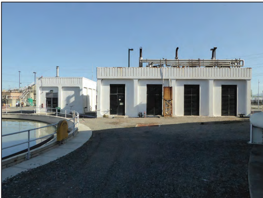
Photograph 29. South side of Buildings 25 and 35; camera facing north, April 21, 2017.
