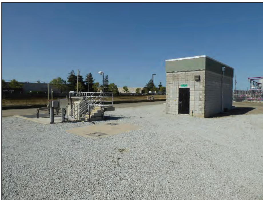
Photograph 54. Building 52 (Final Clarifier Electrical Building); camera facing southwest, April 21, 2017.
