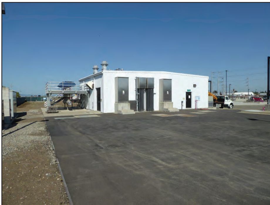
Photograph 34. Building 31 (Aeration Blower Building); camera facing northwest, April 21, 2017.
