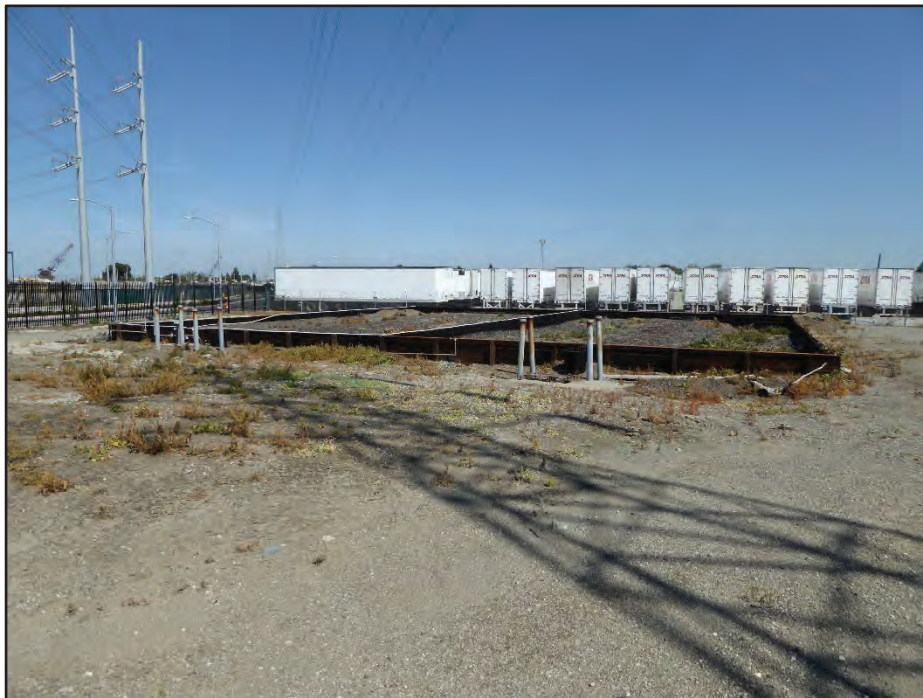
Photograph 51. Structure 49 (Soil Bed Odor Filter); camera facing north, April 21, 2017.
