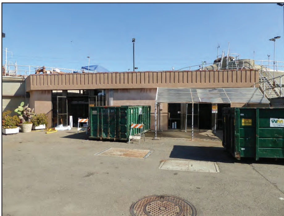
Photograph 23. Building 19 (Equipment Housing Structure); camera facing north, April 21, 2017.
