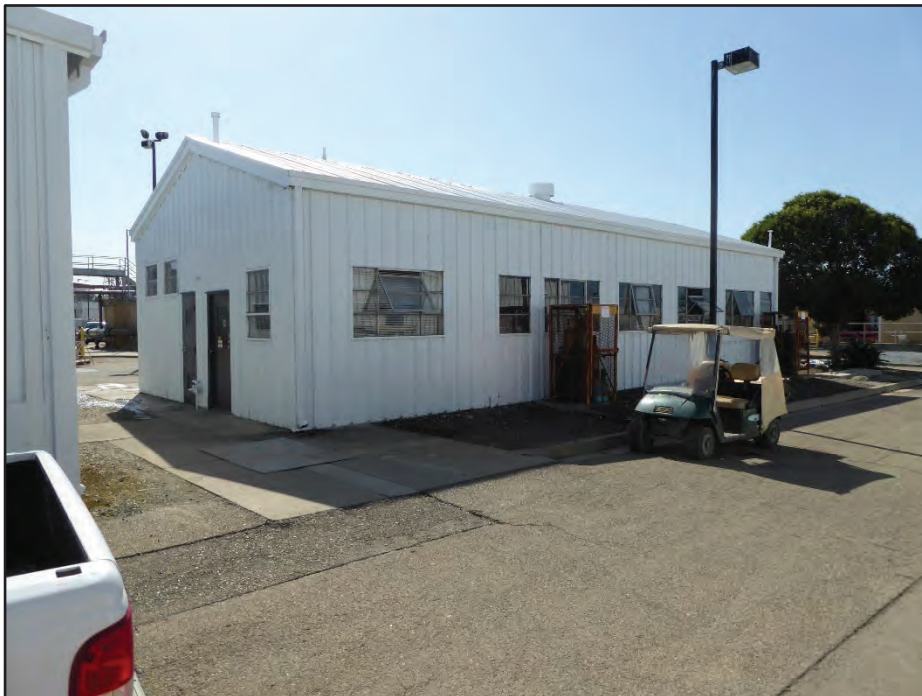
Photograph 17. Building 16 (Storage and Maintenance Building); camera facing southeast, April 21, 2017.
