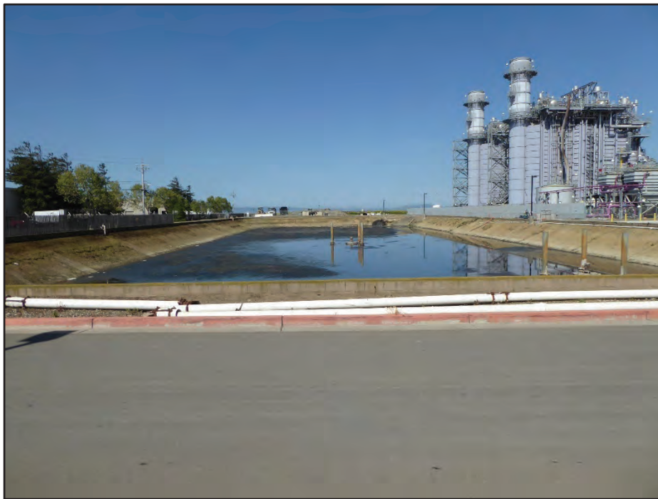
Photograph 10. Structure 10 (Equalization Pond, center) with the neighboring Calpine Energy facility on the right; camera facing west, April 21, 2017.
