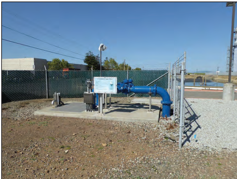
Photograph 53. Structure 51 (Stormwater Pump Station); camera facing west, April 21, 2017.
