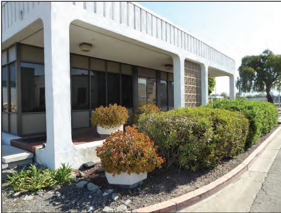
Photograph 20. Detail view of Building 17 façade; camera facing northeast, April 21, 2017.
