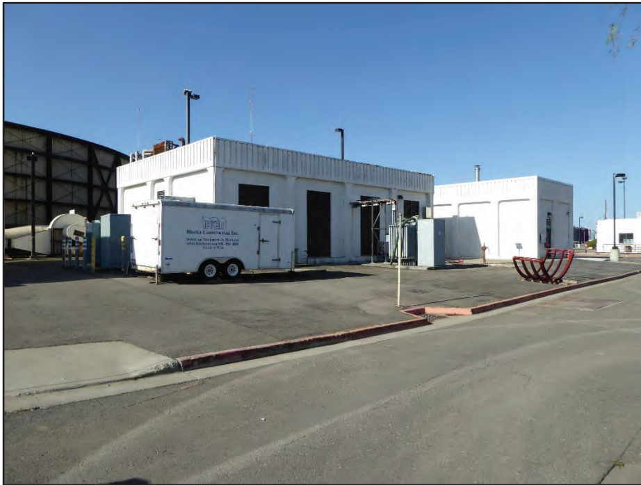
Photograph 28. Building 25 (Old Power Generation Station, center) with Structure 1 (West Trickling Filter, left) and Building 35 (Boiler Building, right); camera facing southwest, April 21, 2017.
