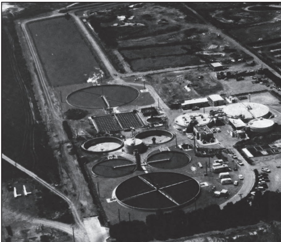
Plate 4: Hayward Wastewater Treatment Plant ca. 1962 – 1970. 20
