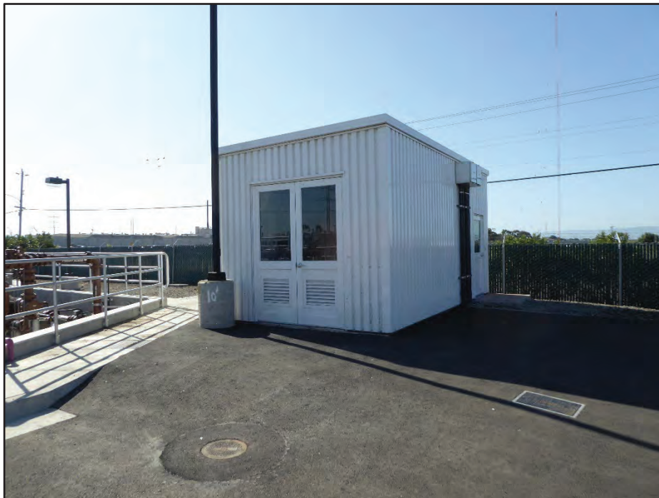
Photograph 25. Building 22 (Chemical Feed Building); camera facing southeast, April 21, 2017.
