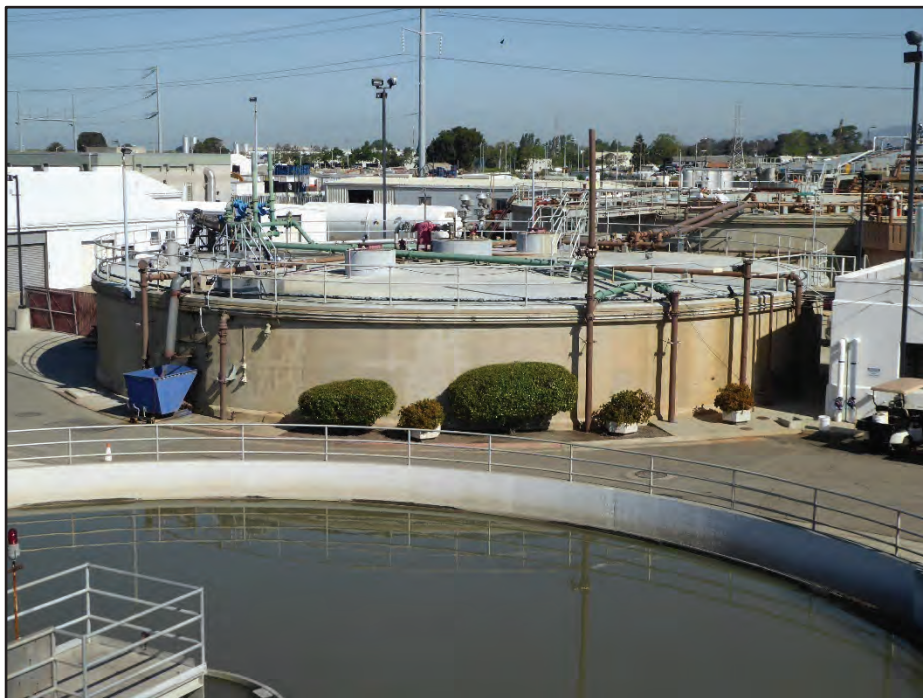
Photograph 7. Structure 7 (Digester No. 3, center), with Structure 4 (Northwest Primary Clarifier, foreground); camera facing northwest, April 21, 2017.
