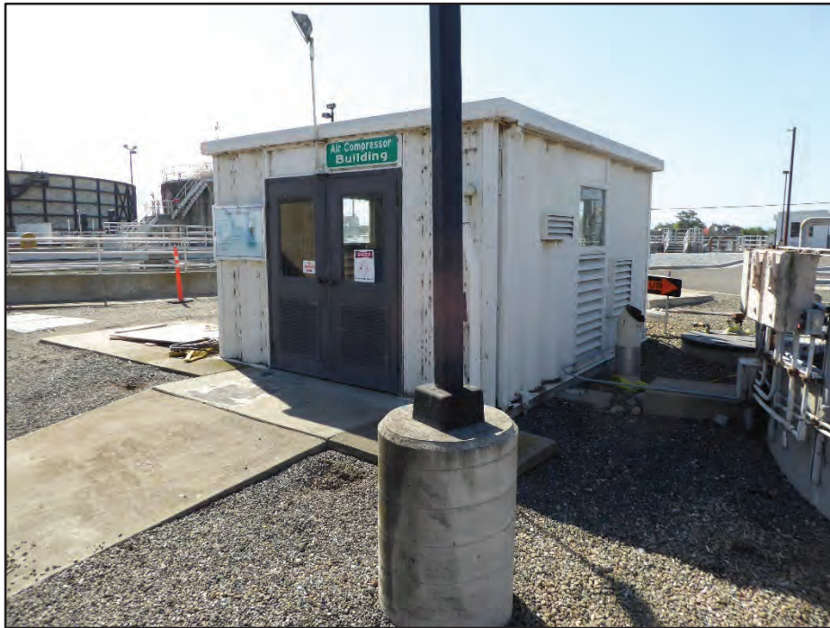
Photograph 24. Building 20 (Air Compressor Building); camera facing southeast, April 21, 2017.
