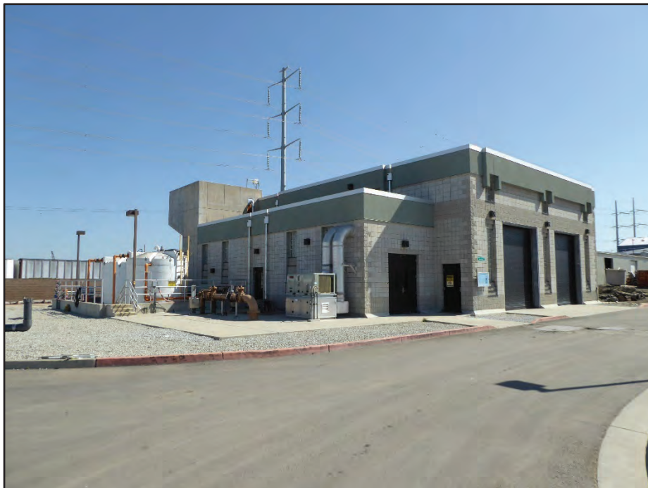
Photograph 47. Building 44 (Solids Thickening Building); camera facing northeast, April 21, 2017.
