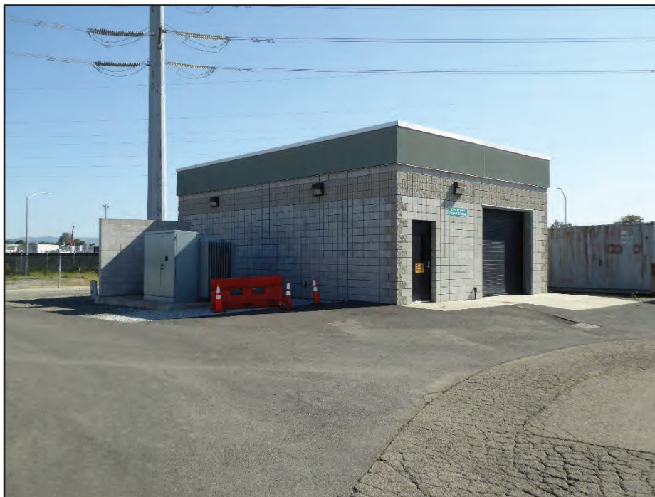
Photograph 43. Building 39 (12kV Import Export Station); camera facing northeast, April 21, 2017.
