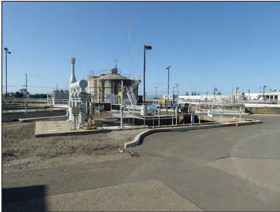
Photograph 12. Structure 11 (Bypass Control Box, center), with Structure 6 (South Vacuumator, center background), Structure 2 (North Primary Clarifier), and Structure 4 (Northwest Primary Clarifier); camera facing south, April 21, 2017.
