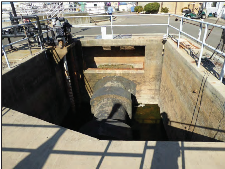
Photograph 13. Detail interior view of Structure 11; camera facing west, April 21, 2017.
