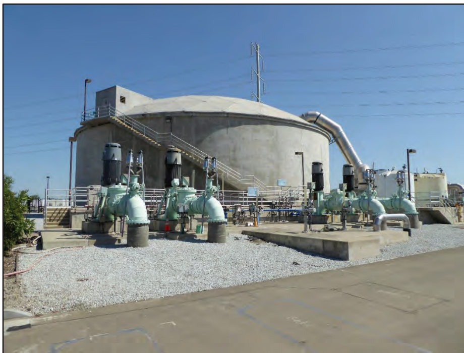
Photograph 44. Structure 40 (East Trickling Filter, background) with Structure 41 (Trickling Filter Pumping Station, foreground); camera facing northeast, April 21, 2017.
