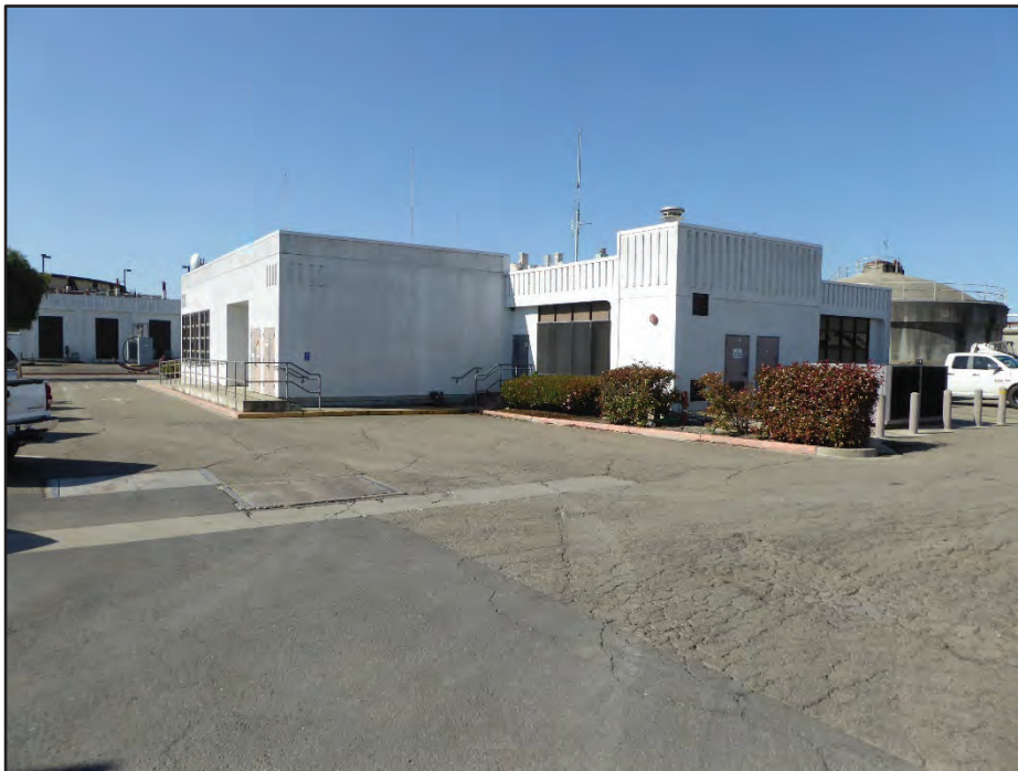
Photograph 21. North and east sides of Building 17; camera facing southwest, April 21, 2017.
