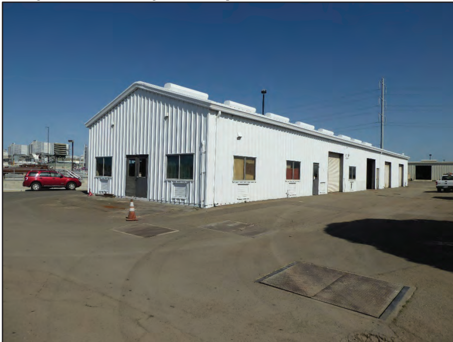
Photograph 31. Building 27 (Maintenance and Electrical Shop); camera facing northwest, April 21, 2017.
