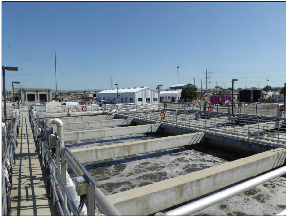
Photograph 36. Detail view of Structure 32; camera facing northeast, April 21, 2017.
