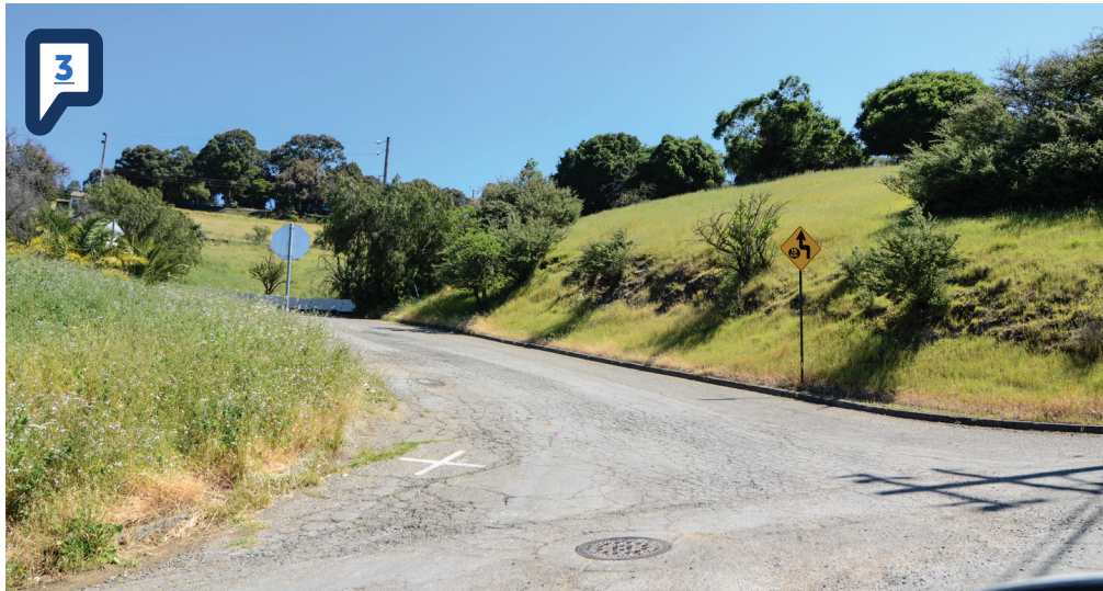
South connection from Central to Maitland
