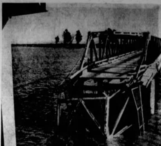
BROKEN SPAN —This gaping hole in the Sacramento River Bridge at Rio Vista was ripped by the Italian freighter Lice during heavy tule fog Sunday. Engineers hope to have a temporary link open for two-way traffic in two to three weeks.—(AP)
