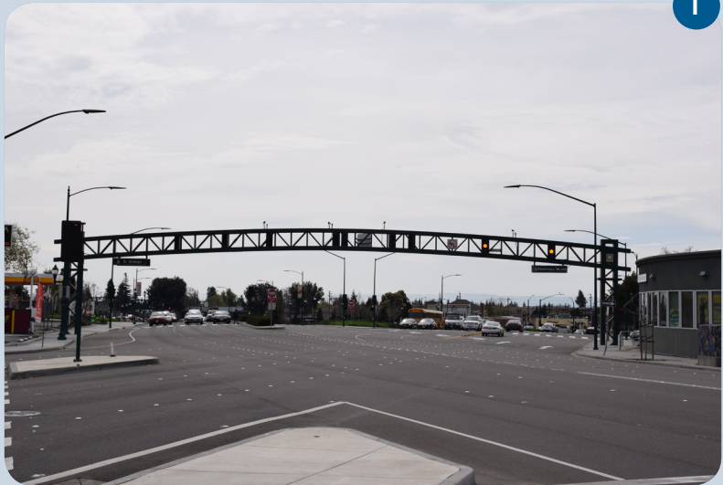
Existing conditions; view looking south at Foothill Boulevard/D Street intersection
