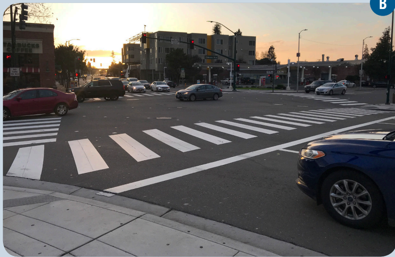
Existing conditions; view looking south at Mission Boulevard/A Street intersection
