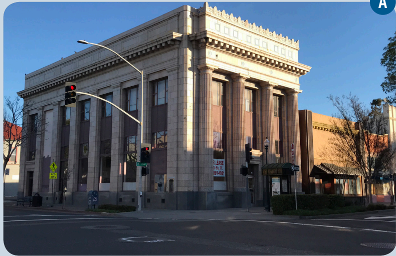
Existing conditions; view looking north at Main Street/B Street intersection
