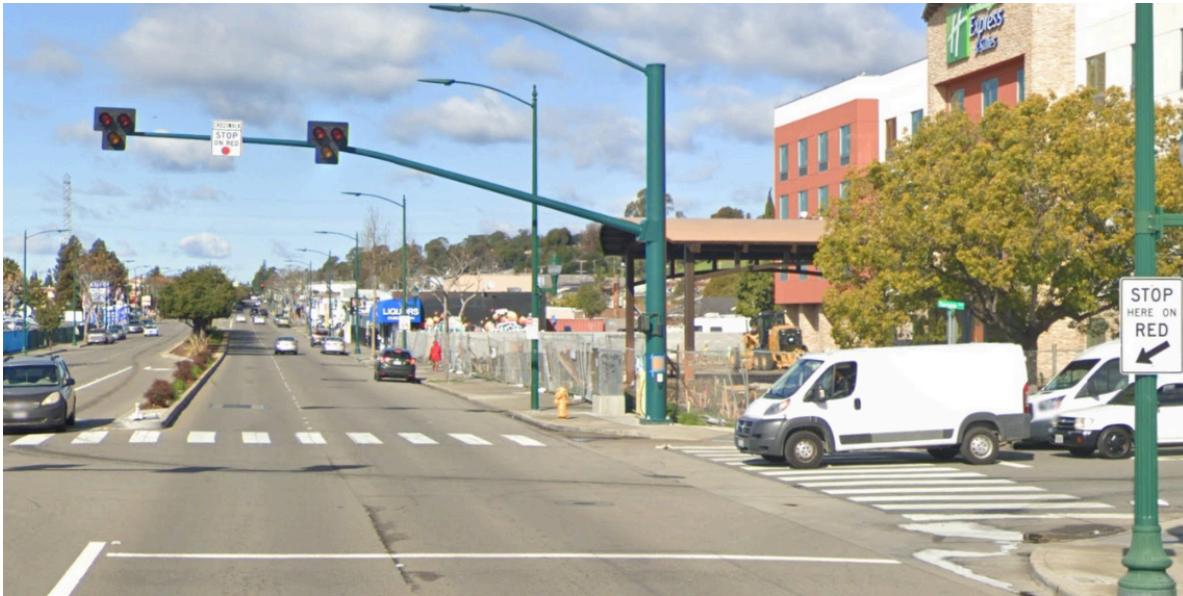
Pictured above is a pedestrian hybrid beacon, also known as a High-Intensity Activated Crosswalk (HAWK) signal, located on Mission Blvd and Torrano Ave. These signals help ensure motorists yield to pedestrians due to their incorporation of flashing beacons.
