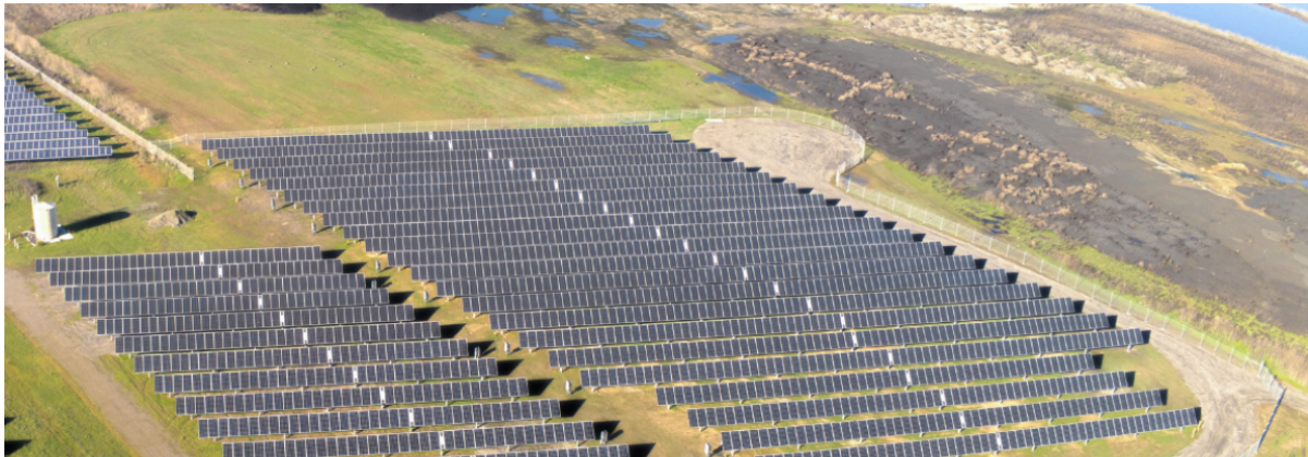
Pictured above is the City's 1.6 megawatt solar photovoltaic system, just west of the Water Resource Recovery Facility (WRRF), formerly Water Pollution Control Facility (WPCF), which has been expanded.
