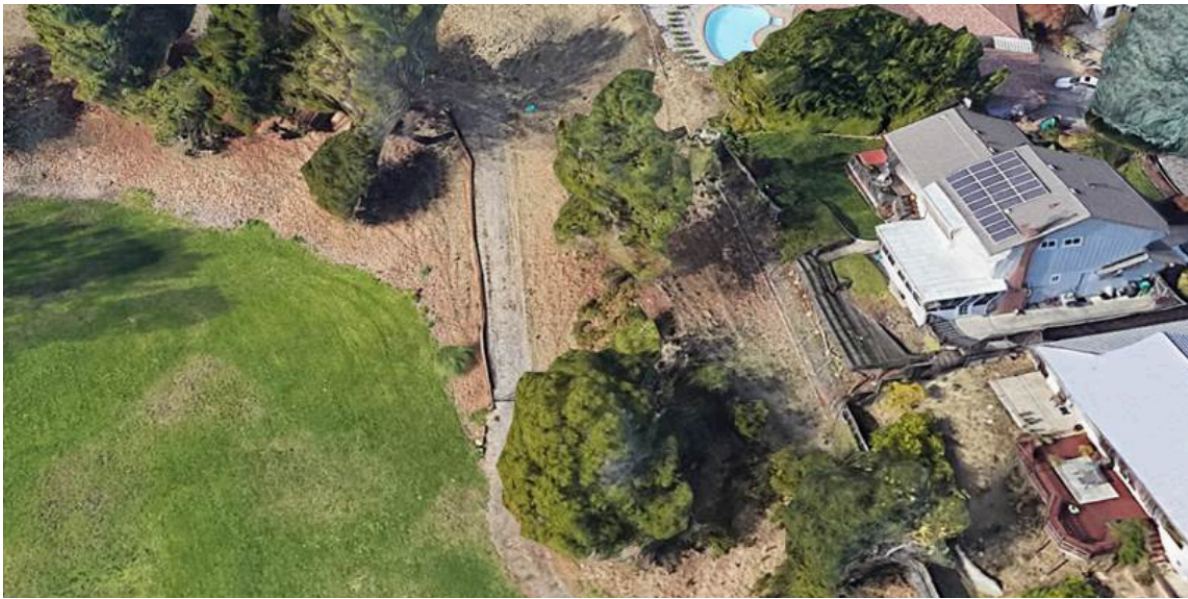
Pictured above is the access road to the Daisy Court sewer easement line.
