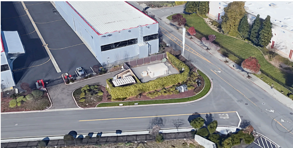
Pictured above in the fence enclosure is the exterior one of the City's 9 lift stations, located at the Hayward Executive Airport. Lift stations move wastewater through segments of the City's sewer infrastructure which rise in elevation, and therefore cannot rely on gravity.
